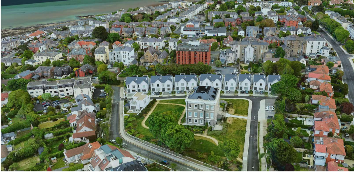
Neptune House (centre) and recent development within curtilage (Google Earth 9.11.21)
