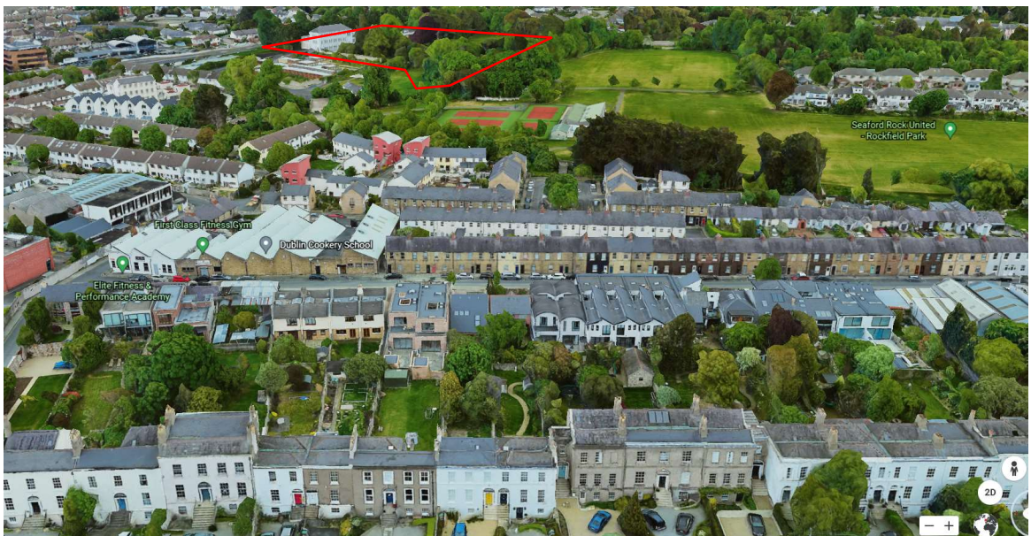
View westwards over Prince Edward Terrace (foreground) towards site (outlined – approximately) (Google Earth 9.11.2021)
