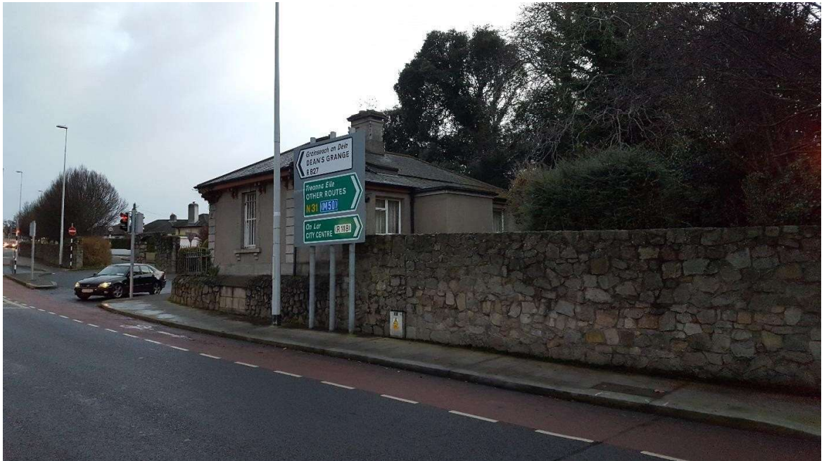
Lodge and lean-to and new boundary wall in un-coursed rubble
