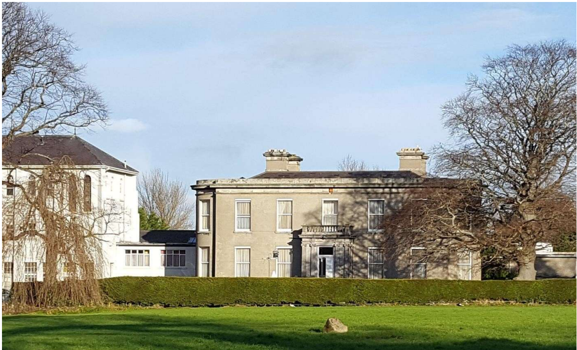
View from South-west (pre-2021)
