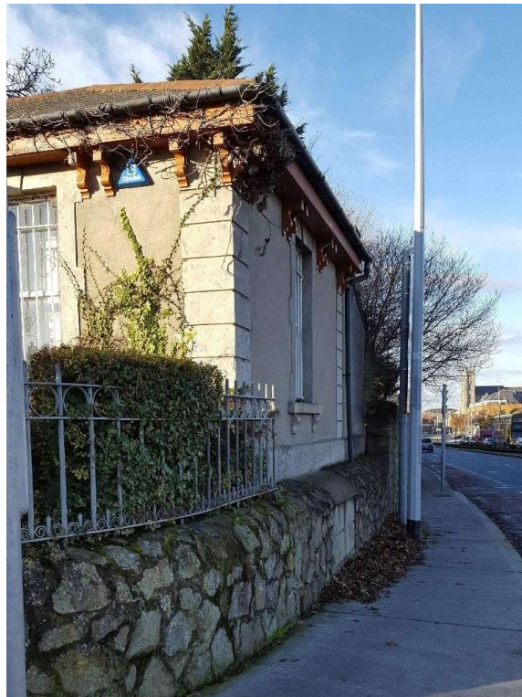
New boundary wall
