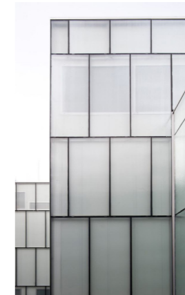
OPAQUE GLASS BACKING PANEL TO PENTHOUSE FACADE
