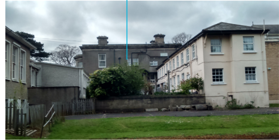
North elevation addressing Temple Road with former structures in place
