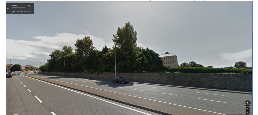
View East up Temple Road with subject lands on right hand side
