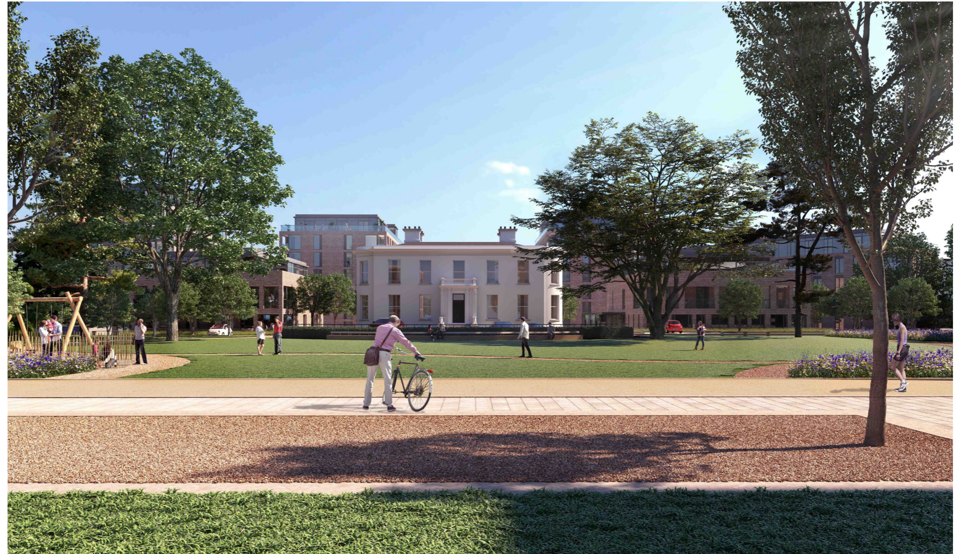
P6 - View from central Parkland towards St. Teresa's House flanked by pavillion blocks C1 and C2
